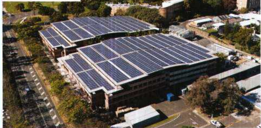
The 1.2MW solar array spans 11 rooftops at the university.
