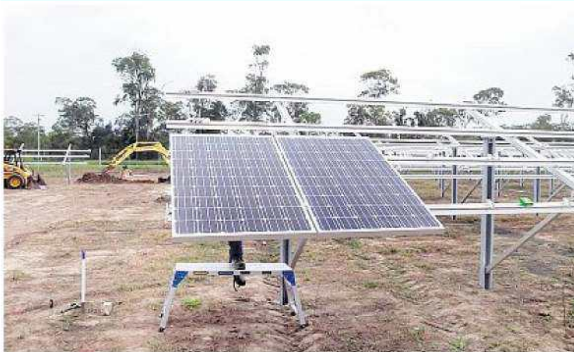
GROUND-BREAKING: The first solar panels installed at Nikenbah solar farm.
