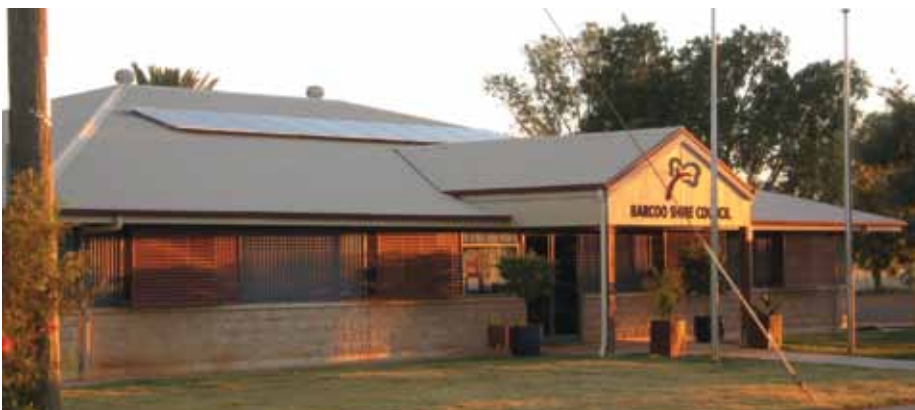
The Barcoo Shire Council Administration Building.
