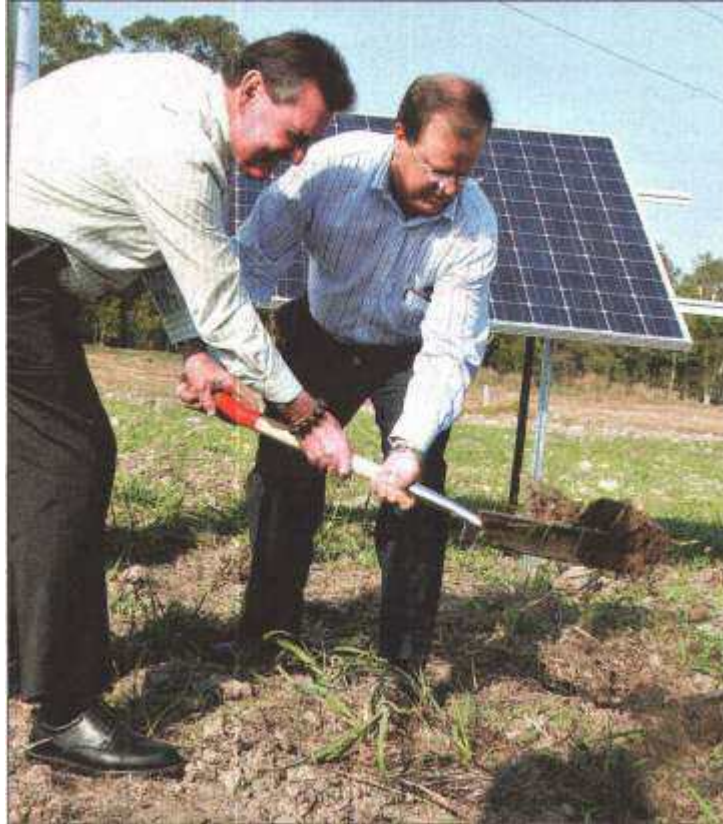
Mayor Mick Kruger and Energy Minister Stephen Robertson turned the first sod at Hervey Bay's $2.7 million solar plant farm on the corner of Boral and Hebblewhite Road at Nikenbah.
