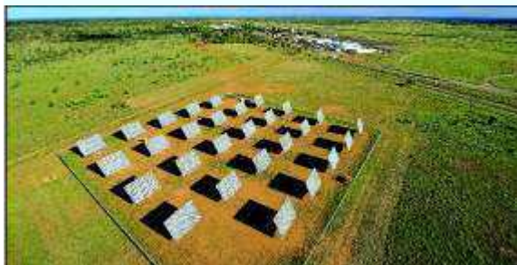
The Alice Springs Airport Solar Power initiative
